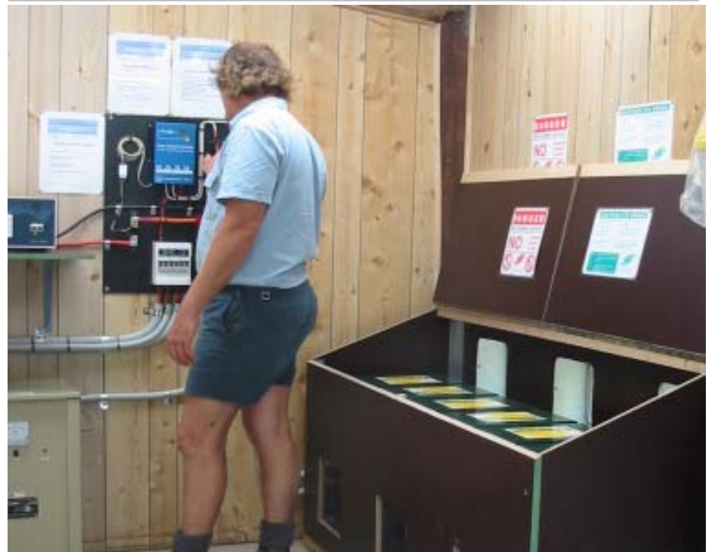
The PL60 Regulator with the regulator, array, charger and batteries fuses.
