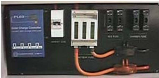
The PL60 Regulator with the regulator, array, charger and batteries fuses.
